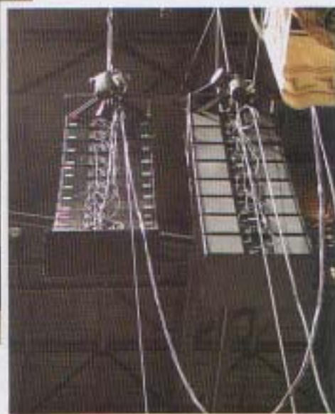
Right, a main MILO array and its companion line of flown subwoofers. Above, one of the arrays for the extreme sides.
