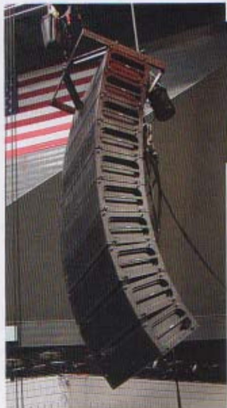
Right, a main MILO array and its companion line of flown subwoofers. Above, one of the arrays for the extreme sides.
